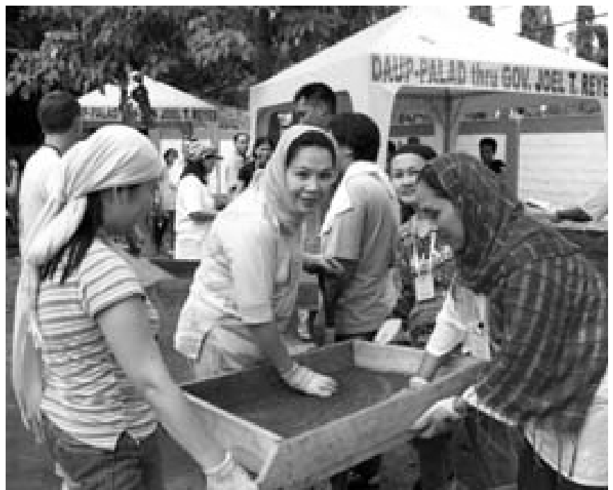
Participants at a workshop in the Philippines learn to sieve the sand used in the construction of the biosand filter.
